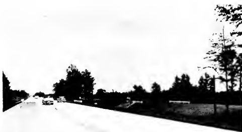
A new section of U. S. 13 south of Salisbury.
